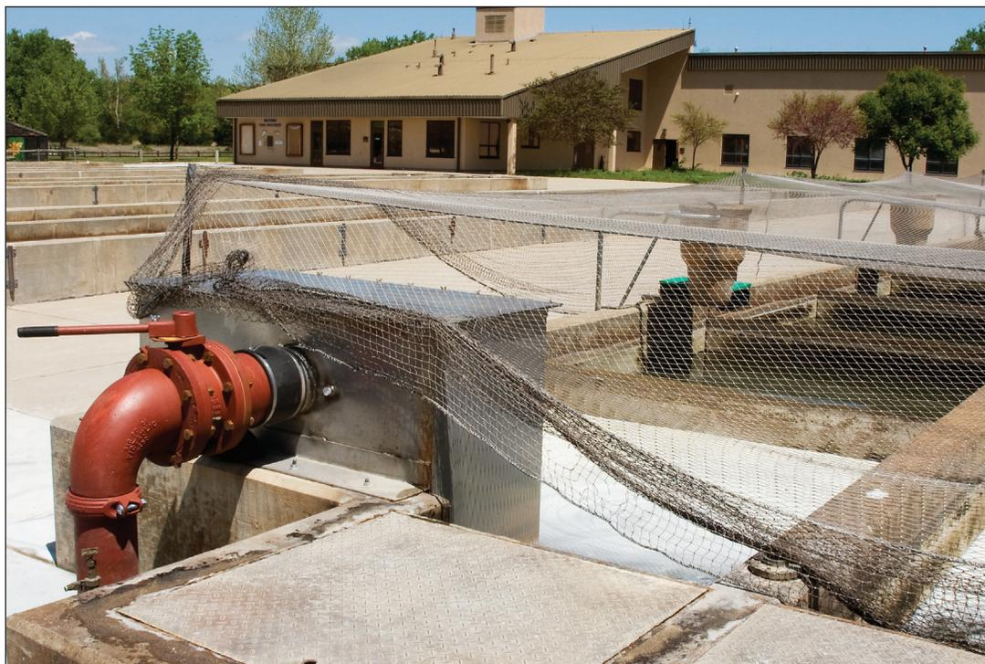
This photo shows a new butterfly valve that feeds water into an oxygen mixing chamber. Controlling water temperature and oxygen content is critical when raising fish in this intensive system.
