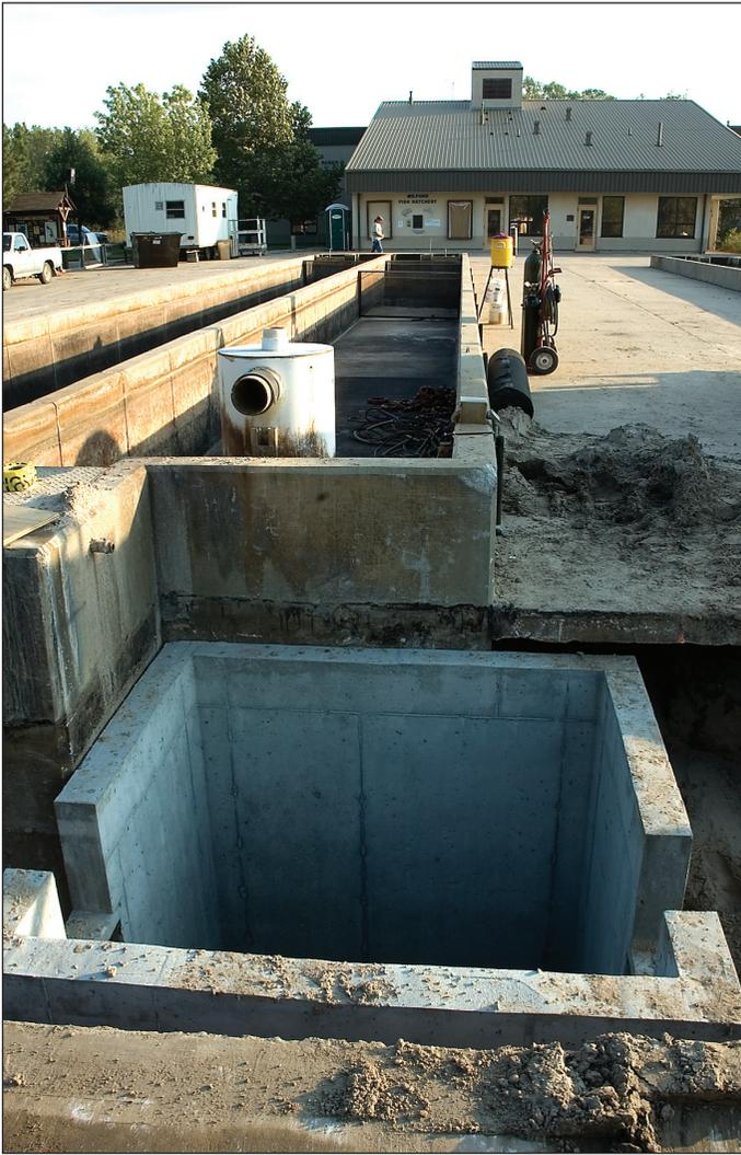
This photo shows a concrete vault that will allow access to water-control valves. Old valves were buried 8-feet deep and could not be accessed for maintenance.
