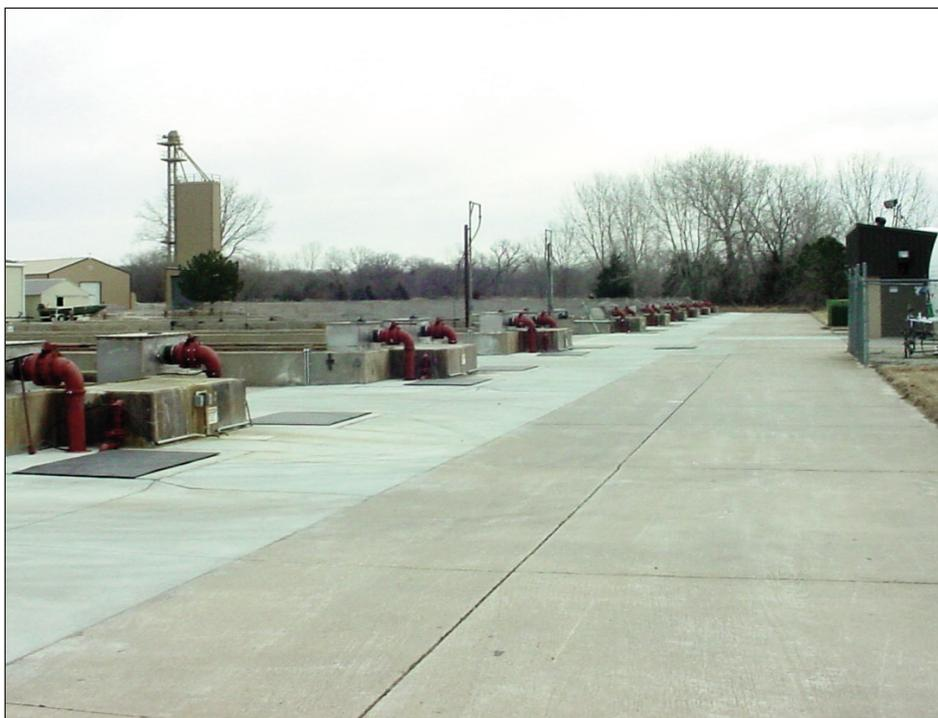
Not only do all race ways have new water-supply lines and valves, but the valves are accessible for maintenance now. The old valves were buried and inaccessible.
